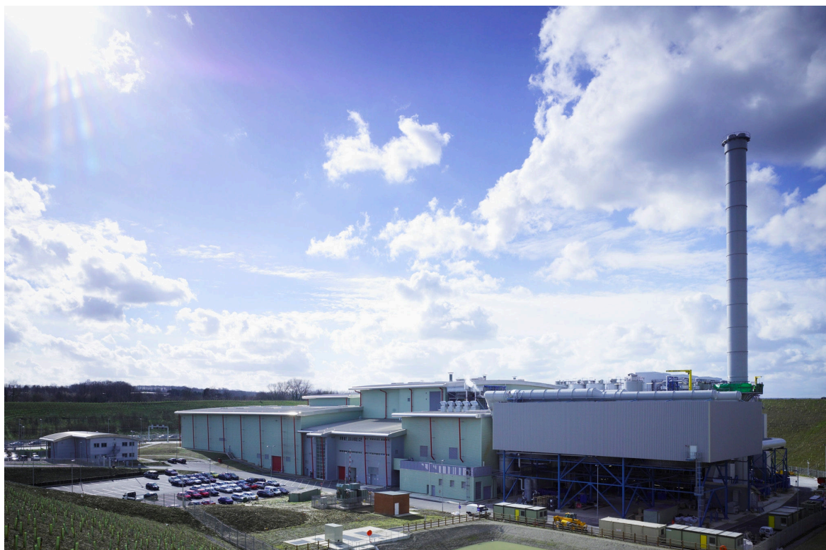
Figure 18: Allington Energy from Waste Plant
